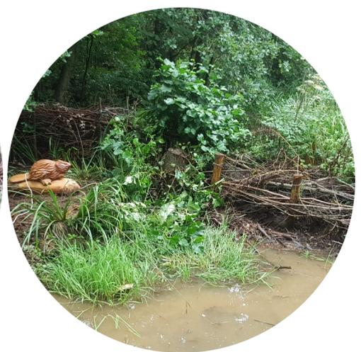
Both small and large dams were used to manage varying flows of water. Smaller flows within Hilbert woods were managed with small scale brush dams. In Grosvenor Park where larger flows were experienced a much larger dam using tree trunks was constructed to slow and retain larger volumes of water.
