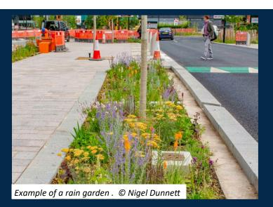
Along the edge of the playground and the car park two rain gardens have been created, these will allow surface water to soak into the ground, preventing the drainage system from becoming overwhelmed during heavy rain.
