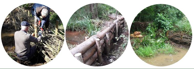
**Both small and large dams** were used to manage varying flows of water. Smaller flows within Hilbert woods were managed with small scale brush dams. In Grosvenor Park where larger flows were experienced a much larger dam using tree trunks was constructed to slow and retain larger volumes of water.
