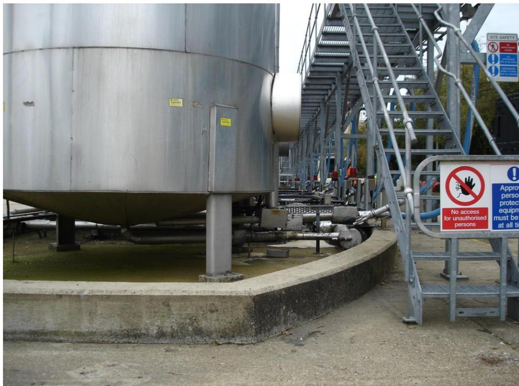
[Figure 10: Concrete bunding surrounding storage tanks](#)
