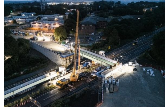
Above: Image of Bridge Beam lift
