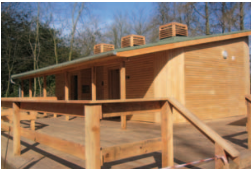
This new amenity block at Trosley Country Park has a number of sustainable construction techniques designed in. It houses office and storage as well as public toilets and Rangers at the park were heavily involved in its design. The building was built using timber felled in the park. Cutaway panels show its construction (below). Mouchel Parkman for KCC
