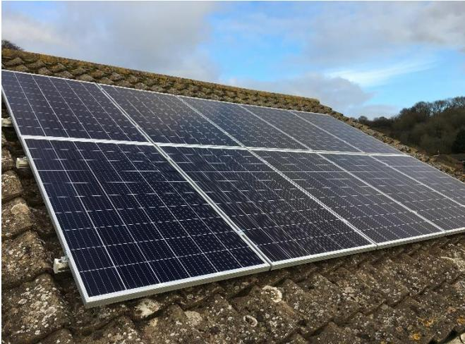
Solar panels generally require little maintenance other than ensuring they are clean to make sure they work effectively. They should last 25 years or more though will likely need the inverter (around £800) replaced at some point. If combined with battery storage this is also likely to need replacing depending on the battery used.
