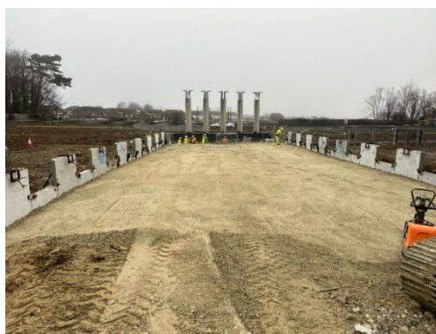
Image above of Wall installation in Section 1B South
