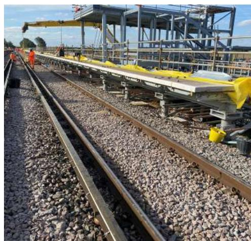
*Installation of platform copers during a line closure.*
