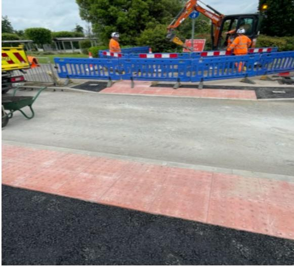
Tactile paving installed for pedestrian crossing
