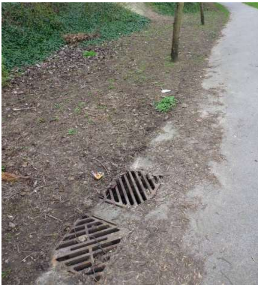
Figure B-2: Sediment likely to have been deposited by a previous overland flow path at Greenhithe Park
