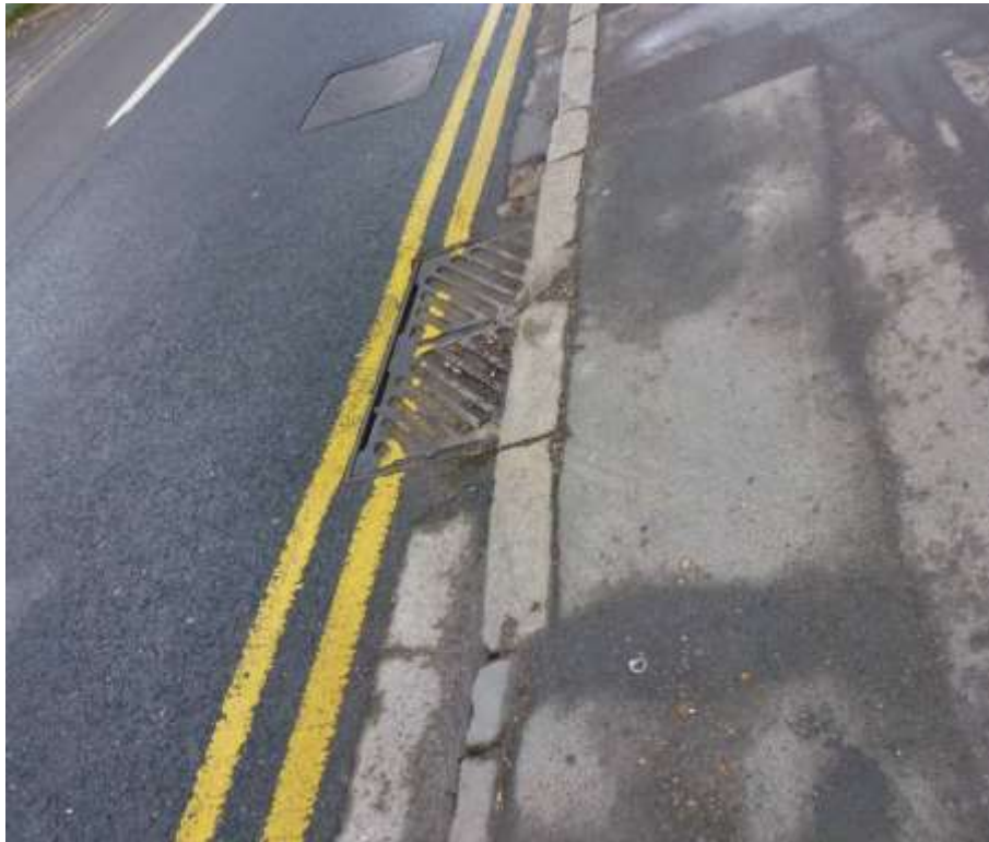
Figure B-5: Blocked gully pots on Hawley Road
