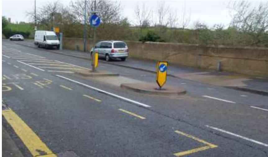
Figure B-14: A concrete wall north of London Road would impound flows on the road
