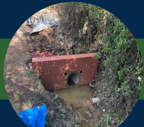
Headwall at the end of the culvert
