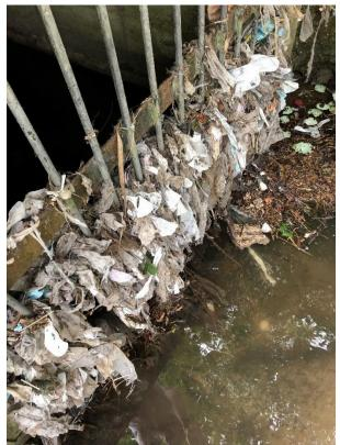
Photo 4 Security screen on outlet of pipe at Saltings Way (18/06/2019)
