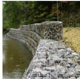
Pre planted coir rolls in combination with a gabion basket terrace will protect the riverbank from erosion whilst the pre planted rolls and seeded gabions will soften the engineered appearance and provide a viewing platform towards Allington Castle.
