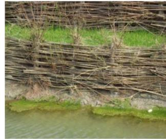
Willow spiling will be used to protect the riverbank from erosion
