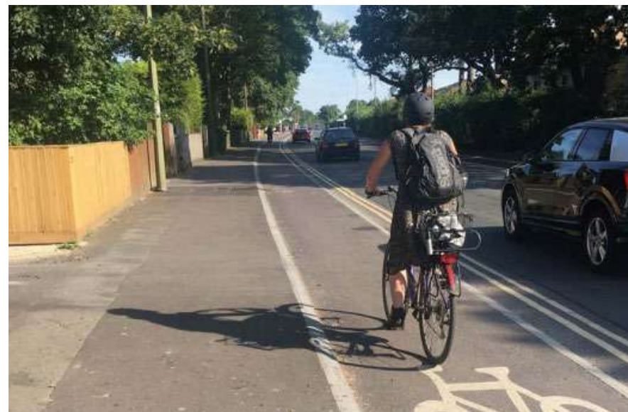
Figure 2: An example of a stepped cycle track. A stepped cycle track is at a different level to both the footway and the road (Source: LTN1/20)
