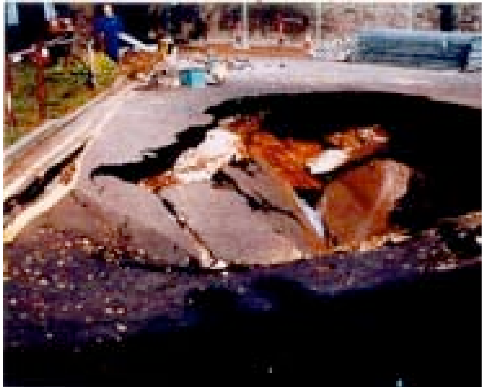
Plate 1 Road collapse caused by washout into gull feature in the Hythe Beds
