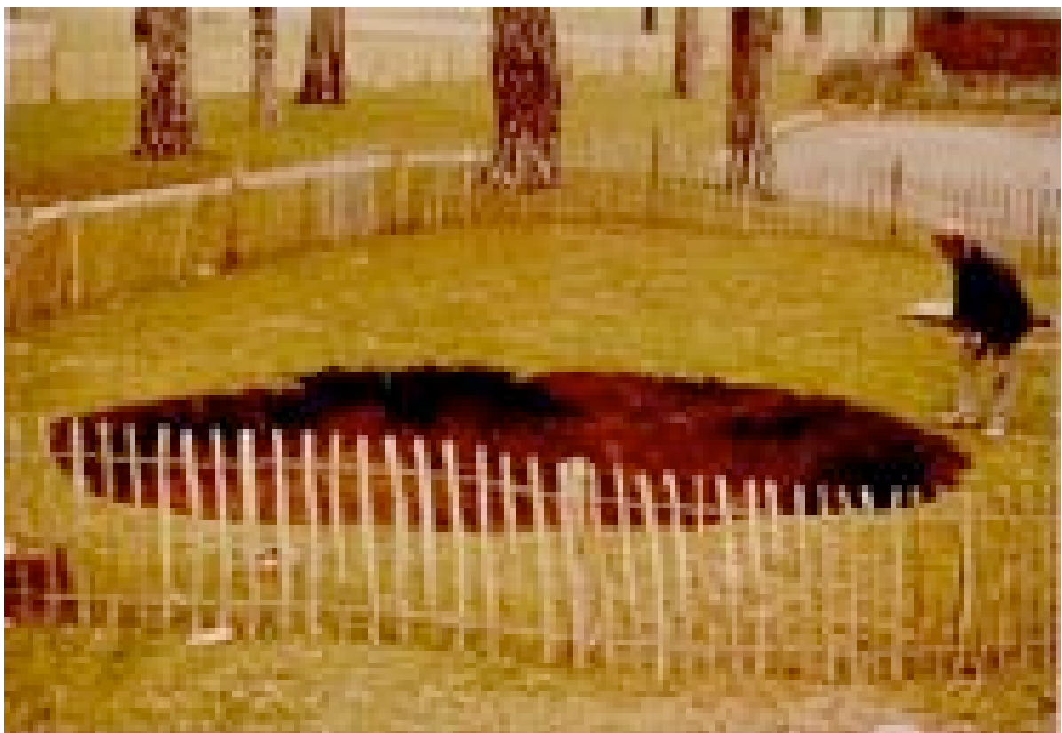
Plate 2 Washout near soakaway in Hythe Beds
