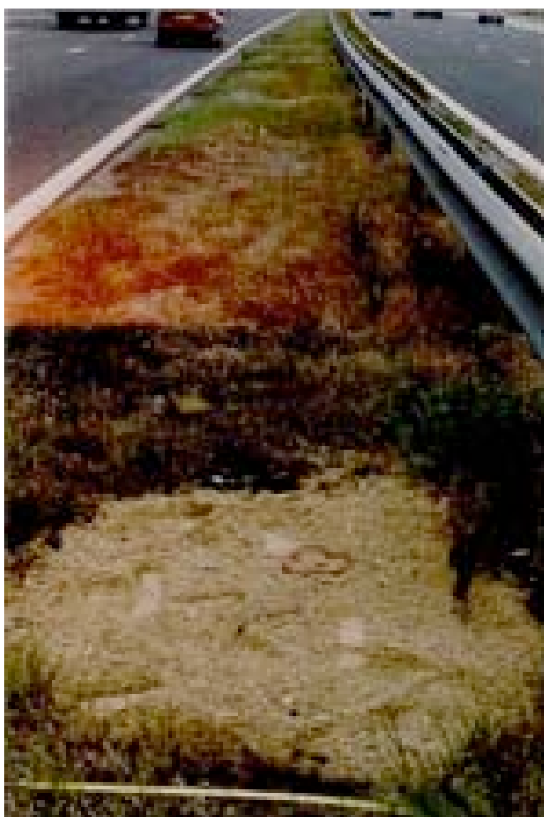
Plate 4 Gravel filled reinstatements adjacent to drain runs over solution features in chalk
