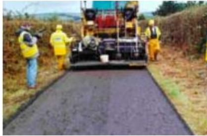
At interfaces between new and existing roads the longitudinal joints in the wearing course must be located outside of the wheel track zone. Ordinarily the surface course will extend to the centre-line or across the full width of the road.
