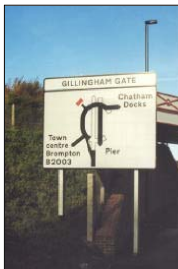
This advance direction sign shows a complicated layout which motorists may have difficulty in understanding (para. 5.6.5).
