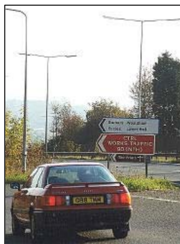
Sign provided without a detailed design. The lettering is far too small for the size of sign
