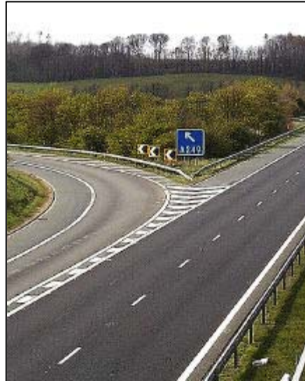
Consideration of re-siting signs and improving conspicuity should be an immediate action where vehicles leave the carriageway regularly.
