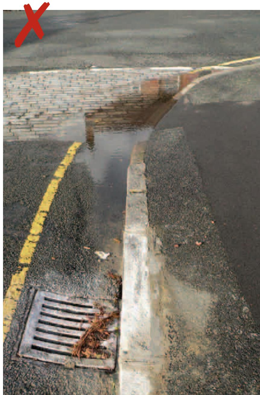
*Road gradients should be designed to avoid ponding in the channel.*
