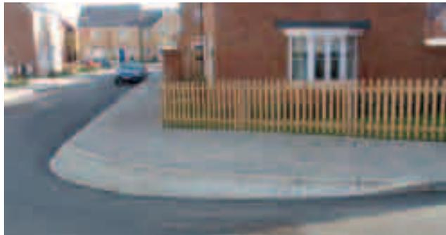
Roads can be widened at bends to allow larger vehicles to negotiate them. Areas that maybe over-run by vehicles can be attractively finished in paving materials.
