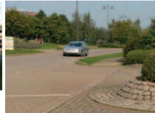
*Industrial and commercial roads designed specifically to take high volumes of traffic need to be designed to be safe as well as attractive. Visibility around bends, junctions and entrances to individual premises must be planned for at the earliest stage of layout design.*
