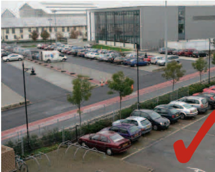
*Parking and access areas for deliveries needs to be considered at an early stage in the design. Each industrial or commercial unit needs dedicated areas for parking that does not conflict with vehicle loading and unloading.*
