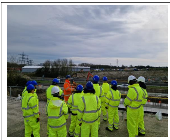
University of Greenwich engineering students on a guided tour of the project site
