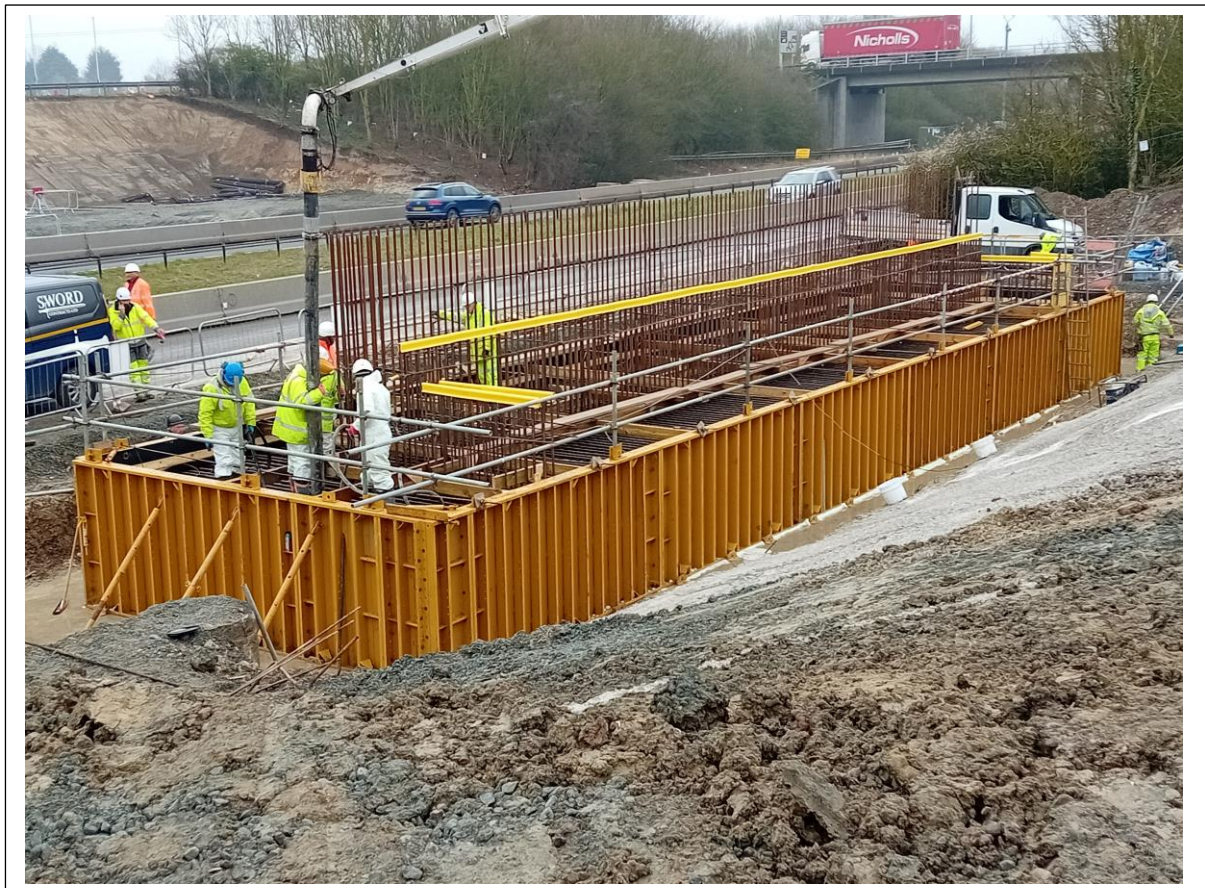
Installation of underground concrete reinforcements for new bridge
