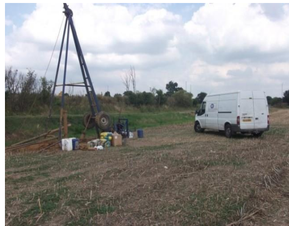
Figure 6 – Example Borehole Rig
