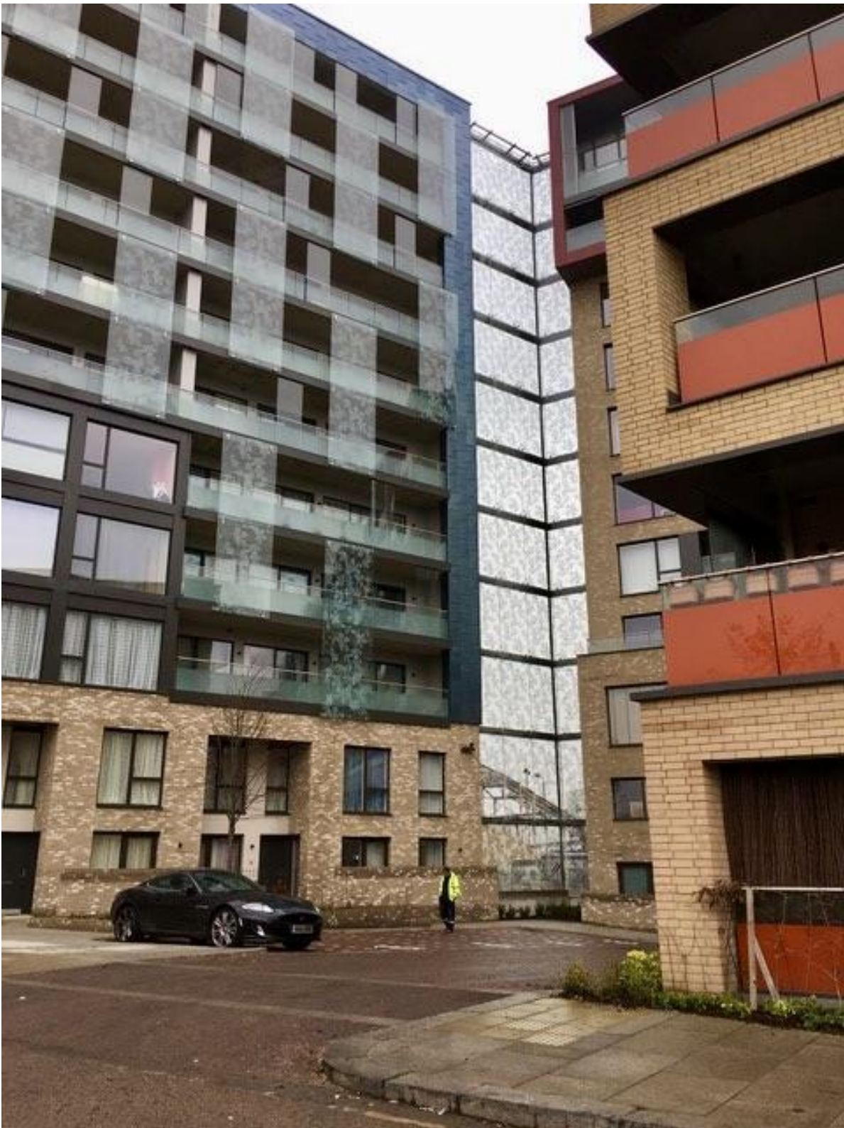
Figure 5 - Noise barrier between buildings installed as part of a new development to mitigate noise from a nearby existing mineral processing facility.
