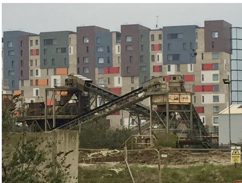
Figure 4 - Examples of new development adjacent to an existing mineral processing facility in Greenwich.
