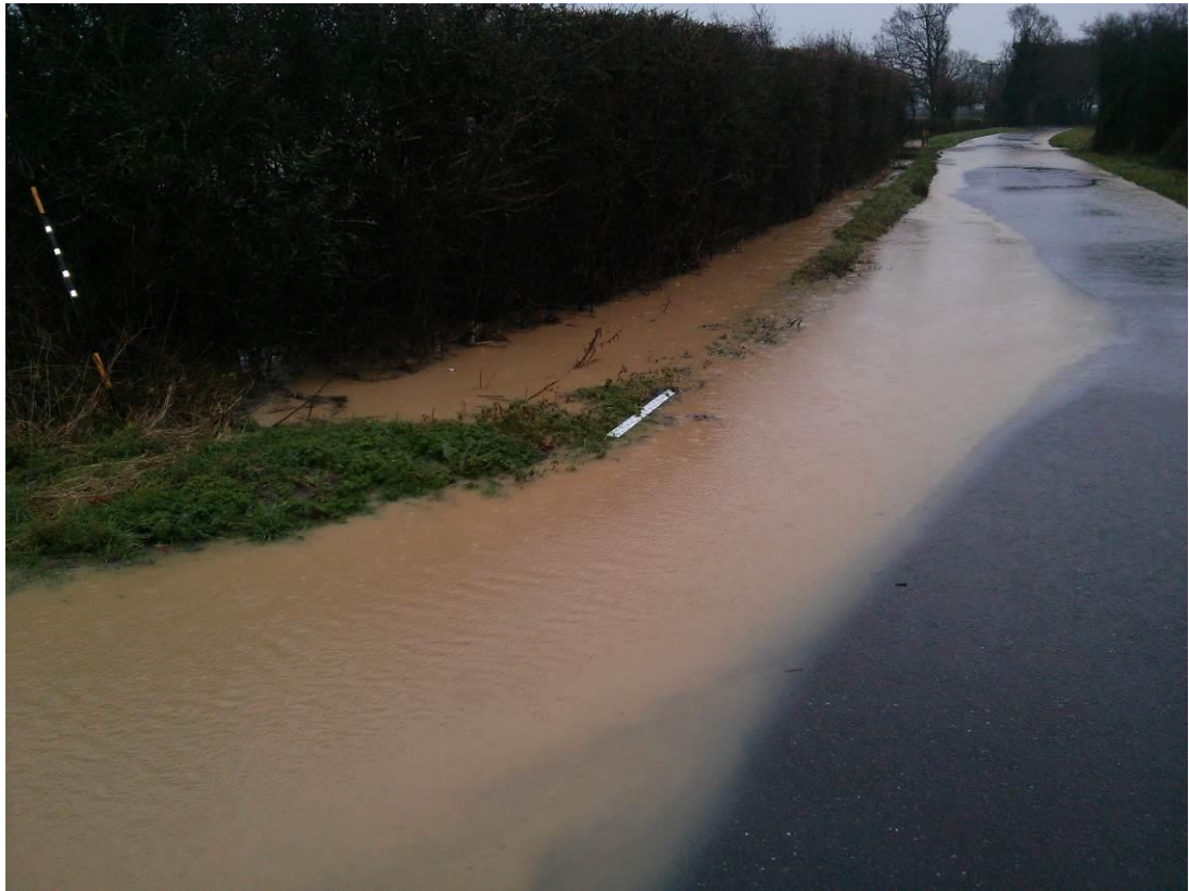
Figure 5. Junction of Bond Lane and Steeds Lane (facing east)
