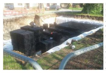
If surface flooding of open areas is not appropriate, the formal drainage system must be designed to accommodate the 100-year storm plus an allowance for climate change. In the case of below ground systems, consultation with the adopting authority will be required if volumes from storms greater than the 1 in 30-year storm are stored below ground.
