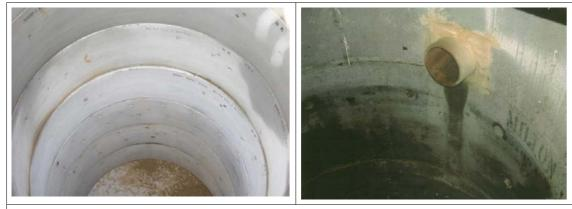
Photos A.1 and A.2 – typical examples of ring soakaways
