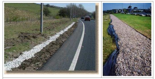
**Photos C.1 and C.2** – typical examples of filter drains, filter drain (left) Filter trench (Source: Susdrain) (right)
