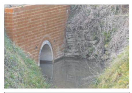
Photo J.1 – Example of a brick headwall
