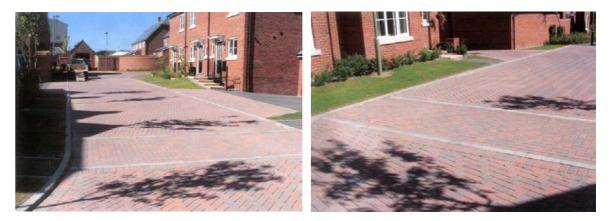
Photos H.3 and H.4 - Permeable paving in a residential development
