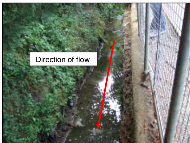
Photo.1: Open channel section – facing south west
