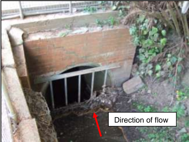
Photo.3: Trash screen in front of culvert inlet (clear)
