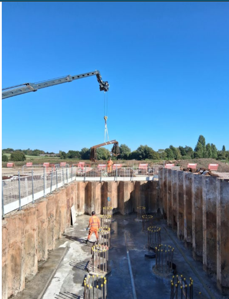
Preparation for pile cap reinforcement
