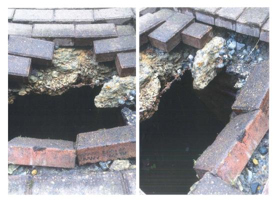
Photo 4 Localised damage to driveway at the downsteam end of the culvert
