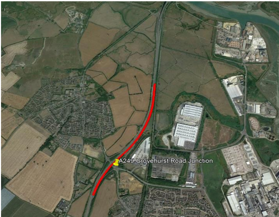
Satellite image showing one running lane due to the southbound traffic management.
