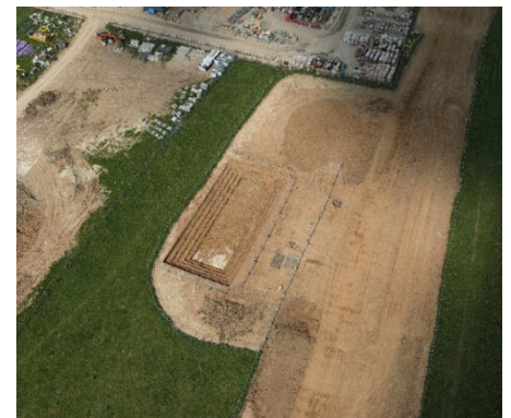
Image: Drone photo of the attenuation tank construction
