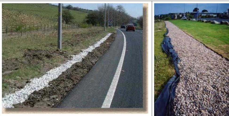
**Photos C.1 and C.2** – typical examples of filter drains, filter drain (left) Filter trench (Source: Susdrain) (right)
