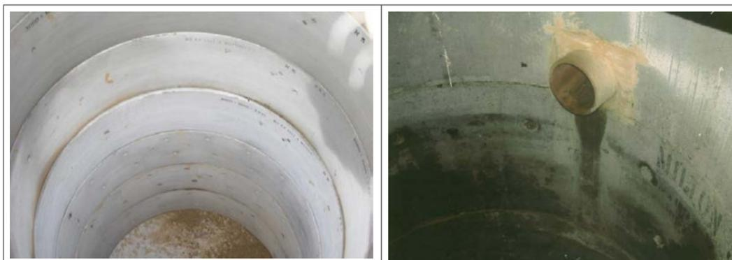
Photos A.1 and A.2 – typical examples of ring soakaways
