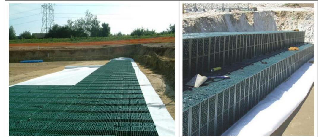
Photos I.3 and I.4 – Examples of different types of Geocellular Unit Installations
