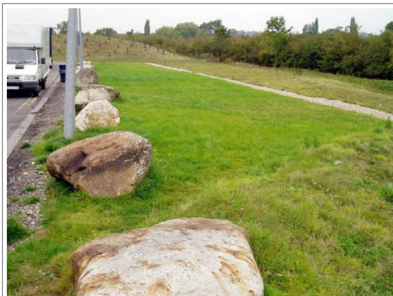
**Photos D.1** – filter strip leading to a filter drain to the right (Source: Susdrain)
