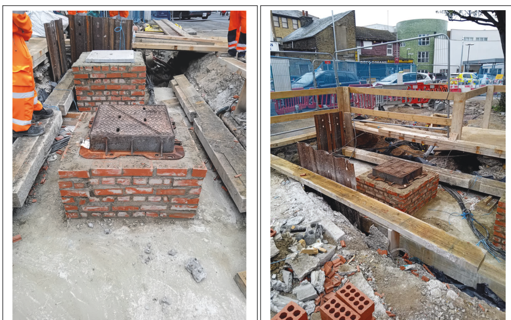
Ongoing works on BT Chamber installation
