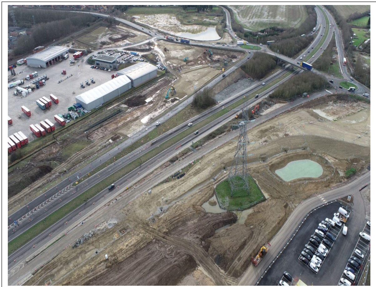
Aerial photo of works progressing on both sides of the A249.
