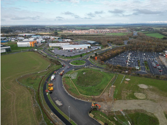
Overhead view of junction at B&Q roundabout Section 2A
