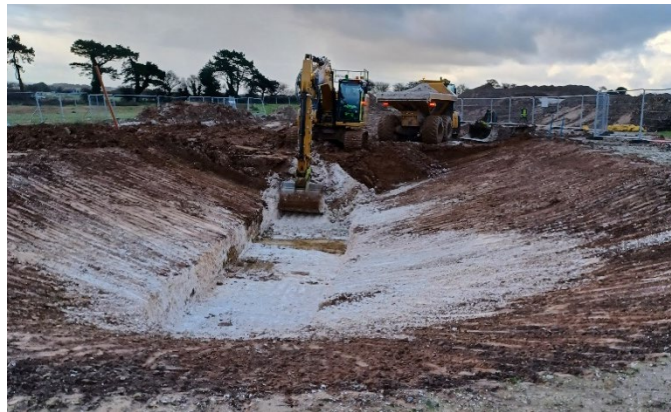
Digging out bio-retention pond
