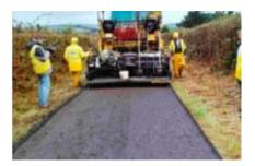
At interfaces between new and existing roads the longitudinal joints in the wearing course must be located outside of the wheel track zone. Ordinarily the surface course will extend to the centre-line or across the full width of the road.
