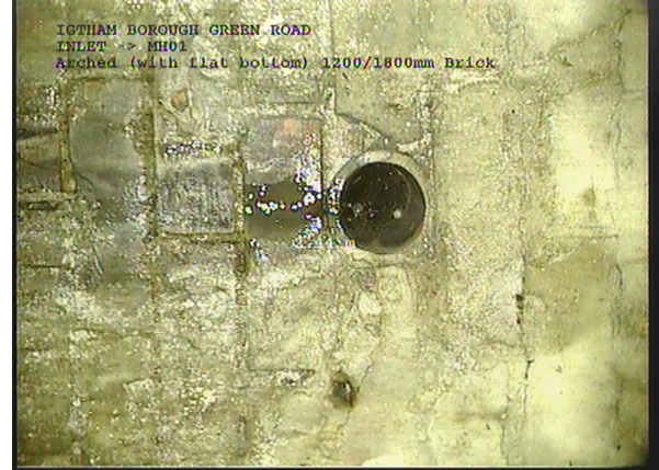
INLETX_d492e8dc-ef9a-45e7-9ac3-ed512f8eeacc_20161114_095241_245.jpg, 00:00:24, 1.51m Junction at 11 o'clock, diameter: 100mm
