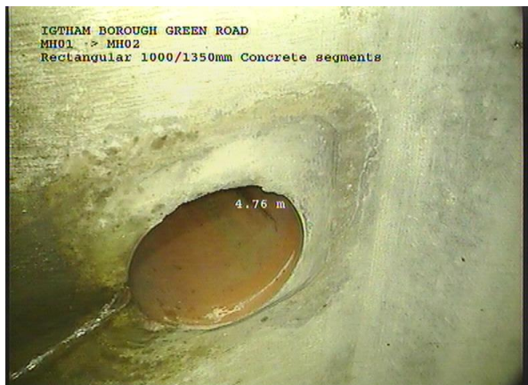
MH01X_b7e2ec72-e2e6-4f4b-b2c2-663589d0c304_20161114_094246_561.jpg, 00:01:07, 4.76m Junction at 09 o'clock, diameter: 300mm
