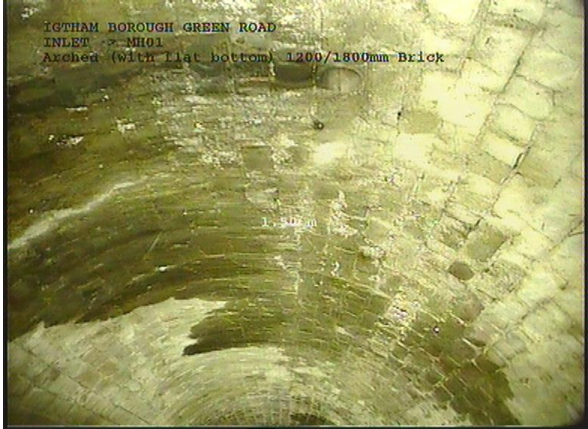
INLETX_a19b43a4-2260-443f-b68c-eb487a443455_20161114_095227_122.jpg, 00:00:24, 1.51m Junction at 11 o'clock, diameter: 100mm
