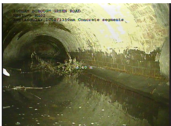
MH01X_6b46b157-8b61-4d00-bb57-7cfaf524f3d9_20161114_094340_165.jpg, 00:01:54, 8.40m Finish node type, manhole, reference number: MH01
