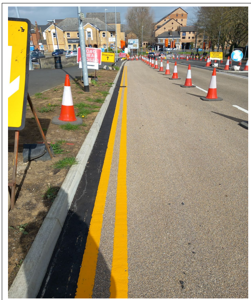
Surfacing and lining works on footpath almost completed.
