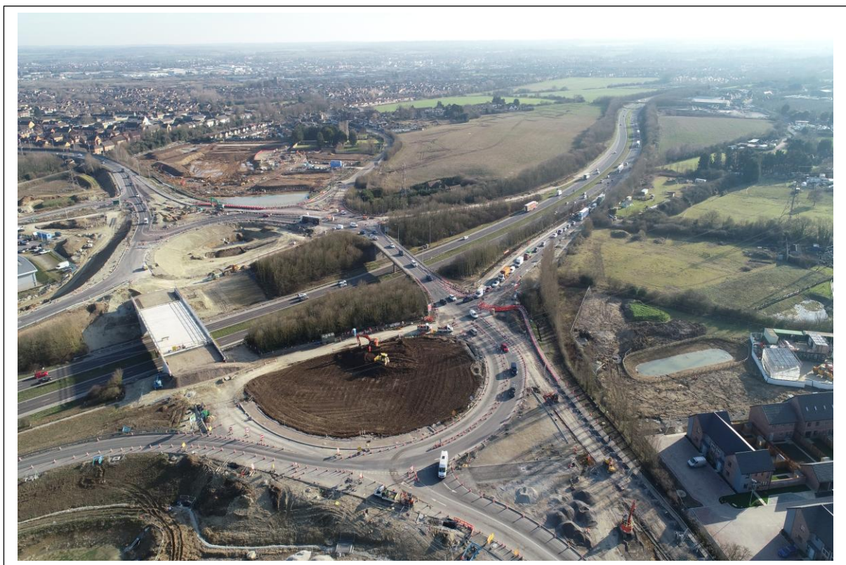
Works in progress at the new Grovehurst Road junction
