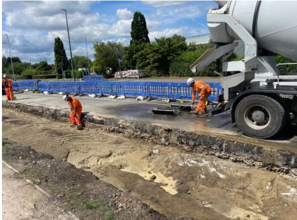
Foam concrete being poured into the Carriageway.
