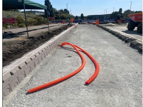
Carriageway backfilled to Type 1 level.
