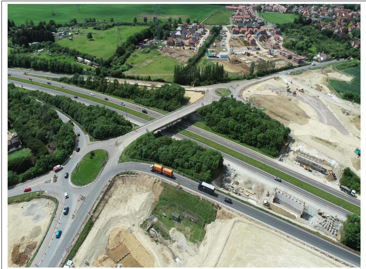
Drone image showing progress of the A249 Grovehurst Road Improvement Scheme
