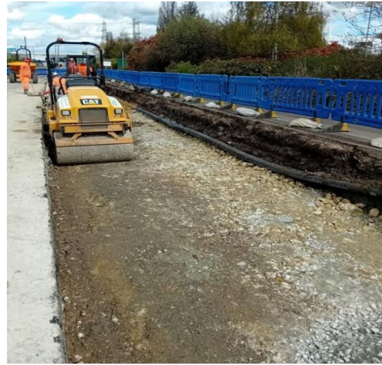
Capping being laid in the southeast verge.
