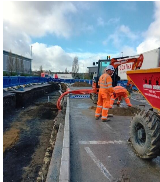
New traffic signal ducts installed.
