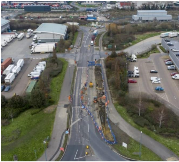
Phase 1 works being carried out at the south.
