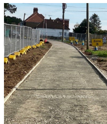
Levelled section of footpath
