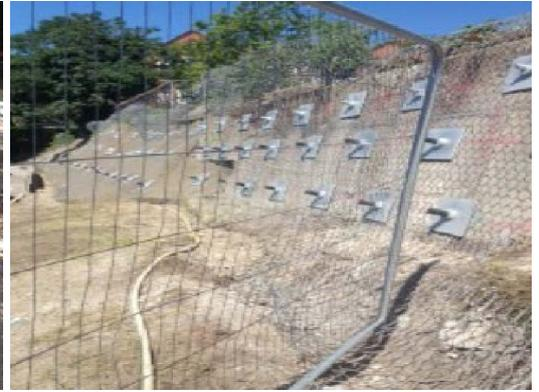
Soil nailing to the embankment
