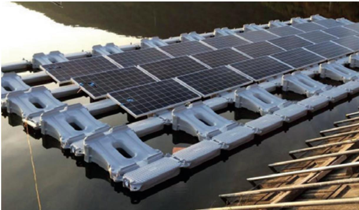
**Floating solar panels and launch ramp.** Source: Floating Solar UK
