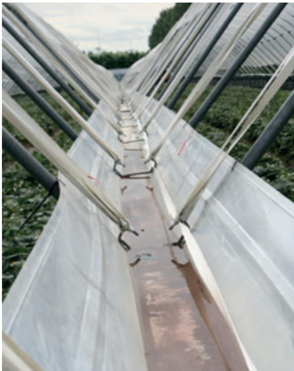
**Gutter system for polytunnel rainwater harvesting.**
