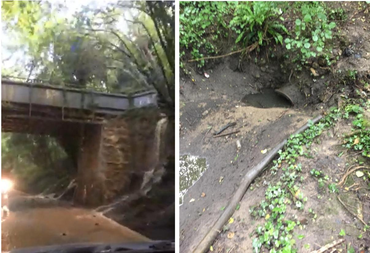
**Photo 6** Out of bank flow adjacent to bridge (left) and view of blocked culvert entrance (right)
