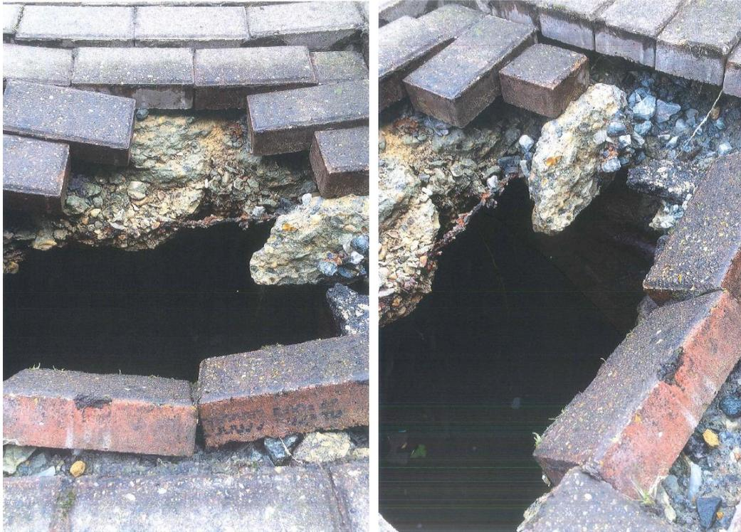
**Photo 4** Localised damage to driveway at the downstream end of the culvert
