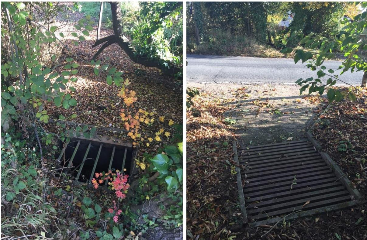
Photo 5 Upstream entrance to culvert (left) and downstream end manhole /road gully
