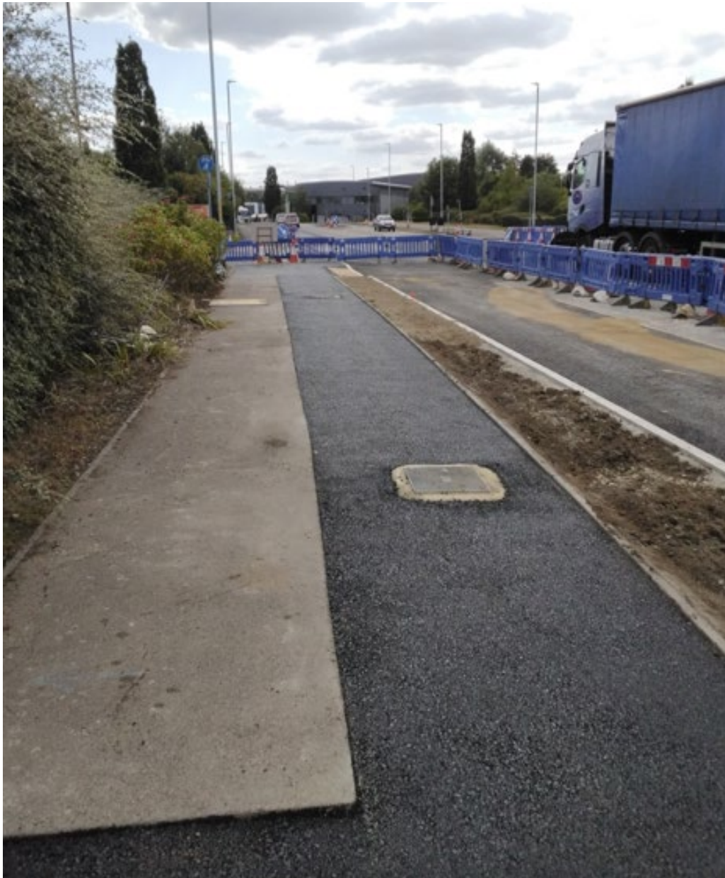
Photo of Rennie Drive northeast footpath reinstatement
