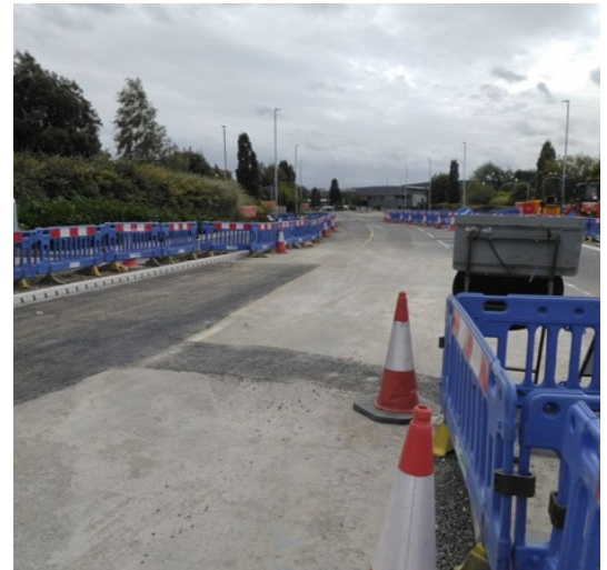
Phase 5 completed binder course
