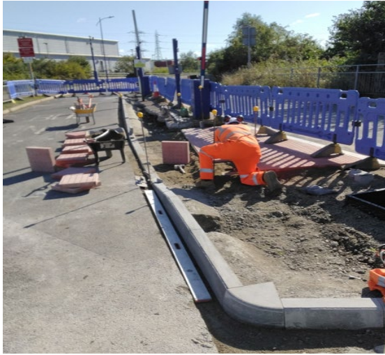
New kerbline and laying tactile paving on Fastway
