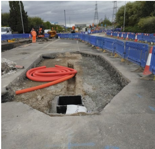
Excavation for new island between
