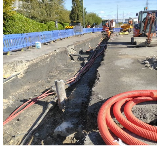
Excavation of road box on west side.
