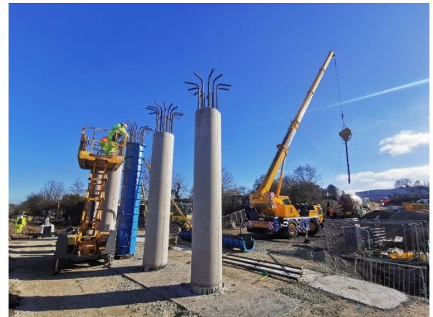
Column Installation - Section 1b South
