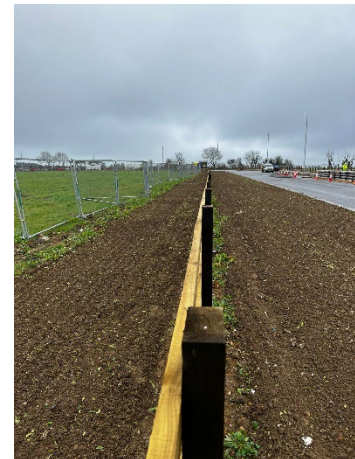
Section 2 landscaping and fencing installation.
