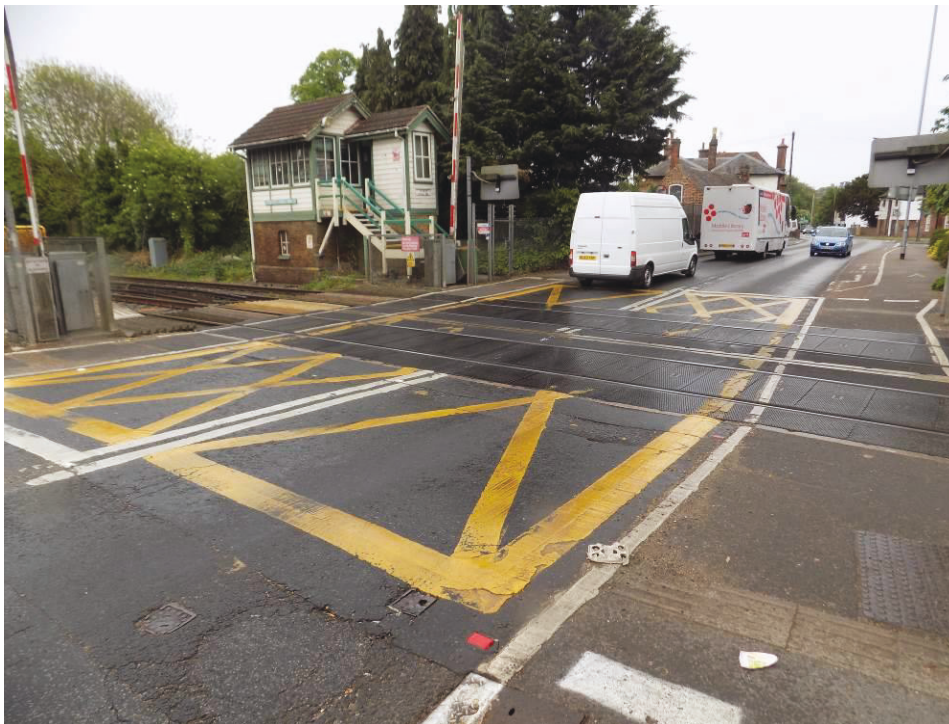
Road Markings - The Hash markings on the crossing itself are faded on the rubber panels (Figure 2.26). Additionally the road markings are faded on approach to the crossing from the south side (Figure 2.27 and 2.28), and slightly faded on the approach to the crossing from the north side (Figure 2.29 and 2.30)
