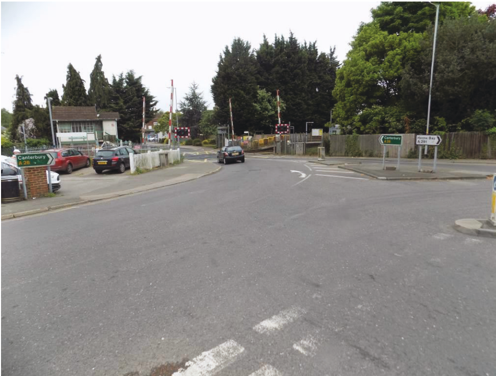
Figure 2-29 - Faded Road Markings on Distant Approach to North Side of Crossing
