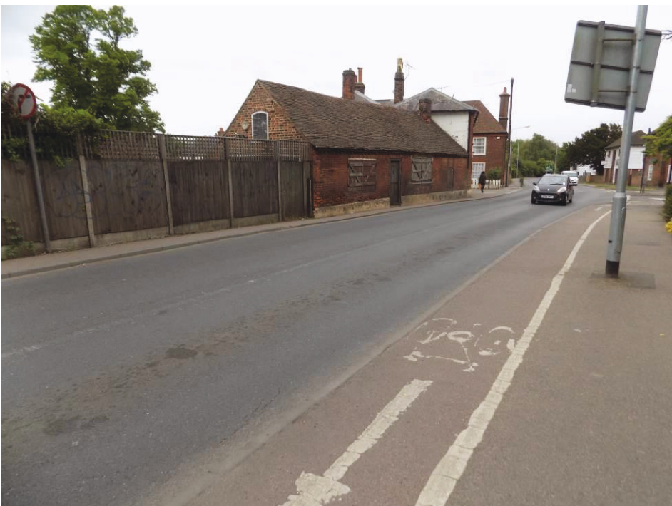
Figure 2-28 - Faded Road Markings on Distant Approach to South Side of Crossing
