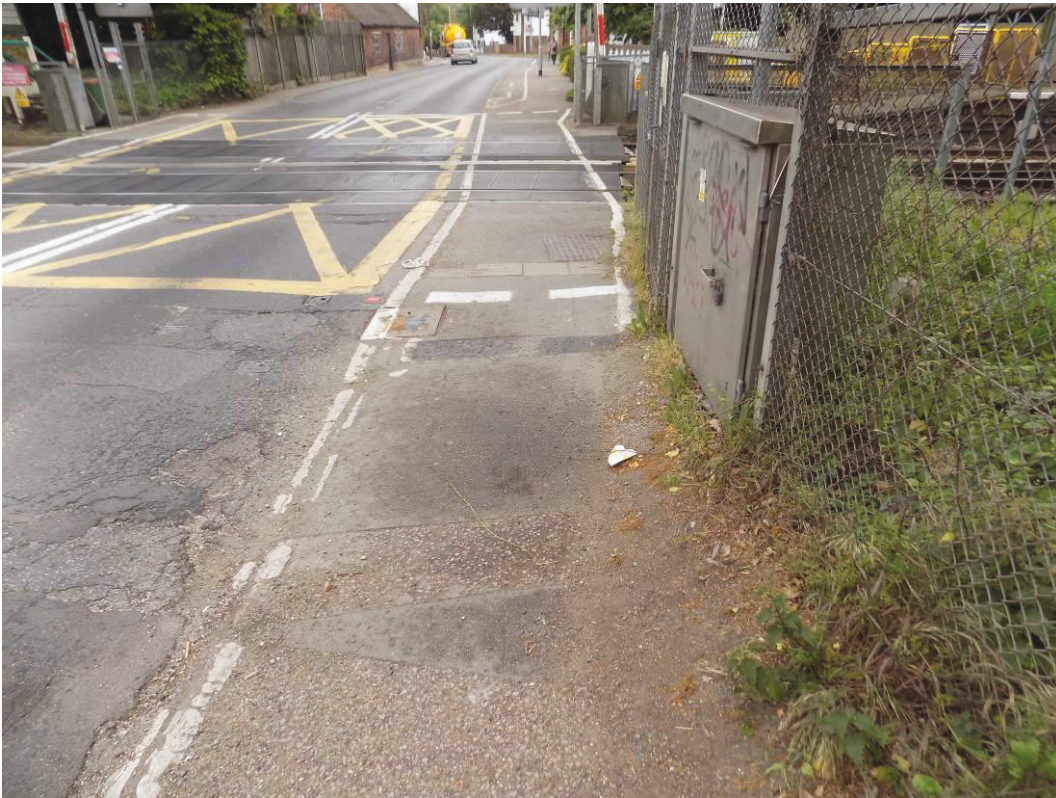
Figure 2-7 - Footway Over Crossing (West Side). Note Uneven Approach to Crossing
