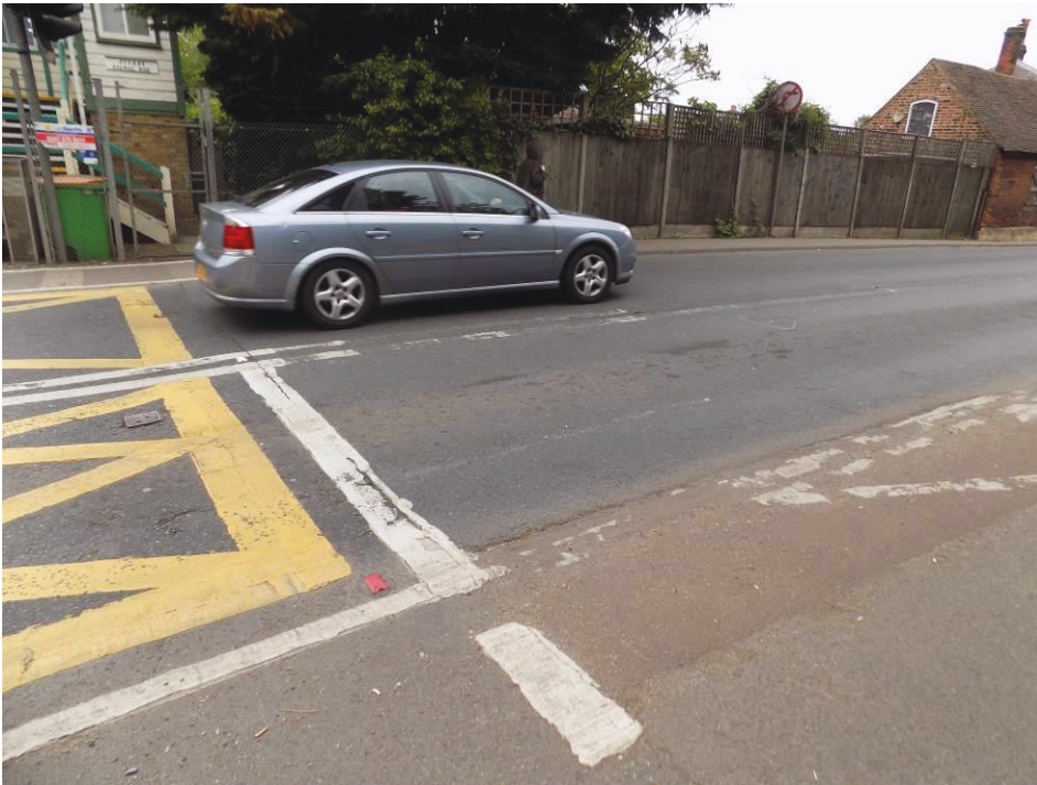
Figure 2-27 - Faded Road Markings on South Side of Crossing
