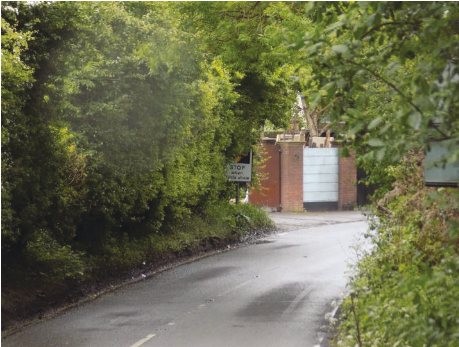
Figure 2-30 - Obscuration of Warning Sign on North Approach
