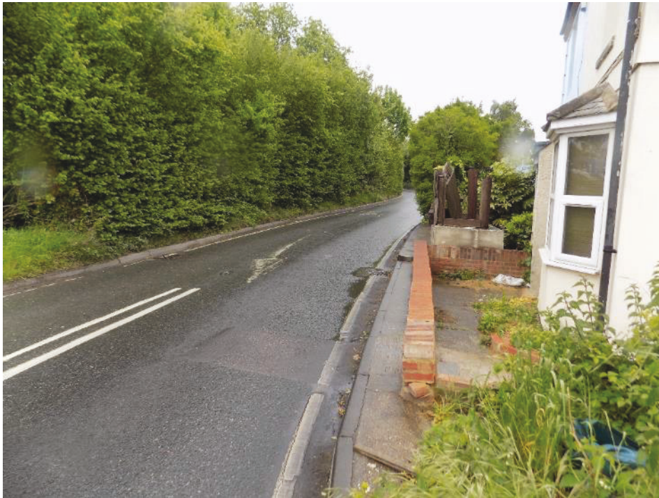
Figure 2-28 - Faded Road Markings on North Approach to Crossing (2)
