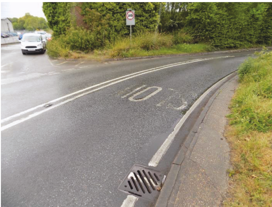
Figure 2-27 - Faded Road Markings on North Approach to Crossing
