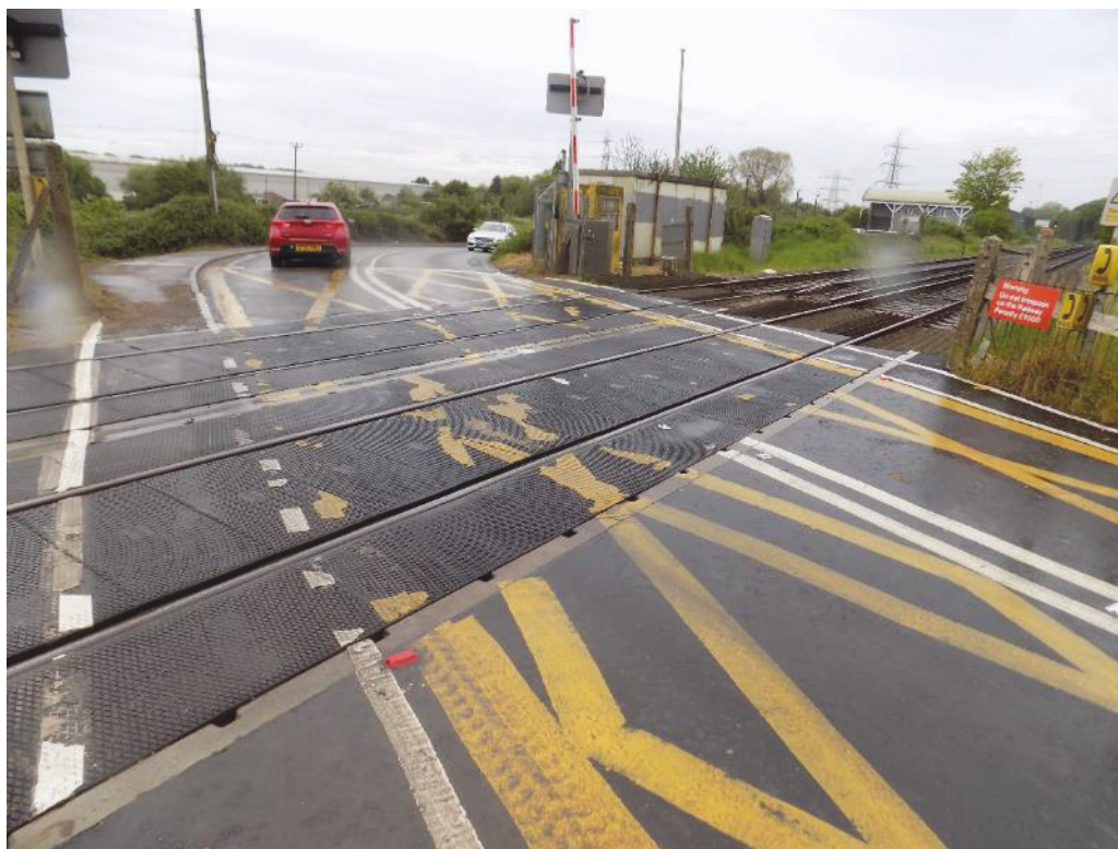
Figure 2-24 - Faded Hash Markings on Crossing
