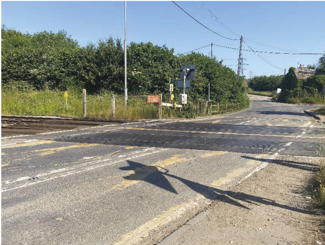
Figure F-12 – Level crossing decking
