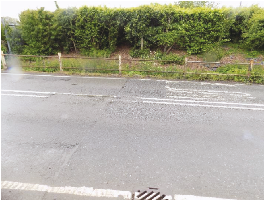
Figure 2-26 - Faded Road Markings on Close Approach to Crossing (North Side)
