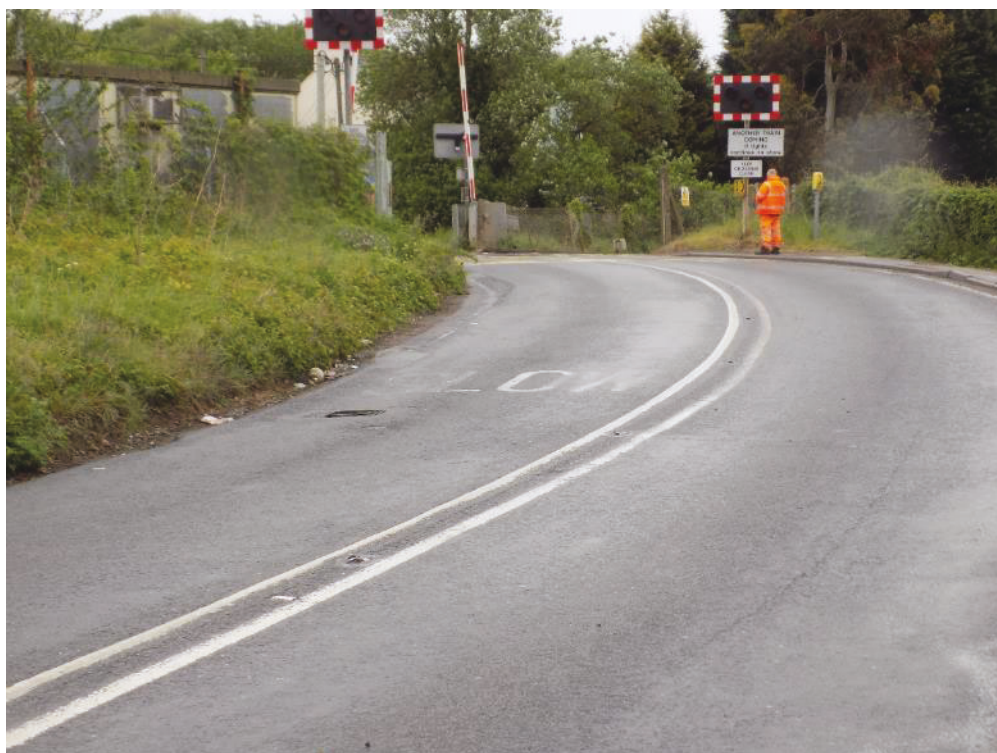
Figure 2-25 - Faded Road Marking on South Approach to Crossing
