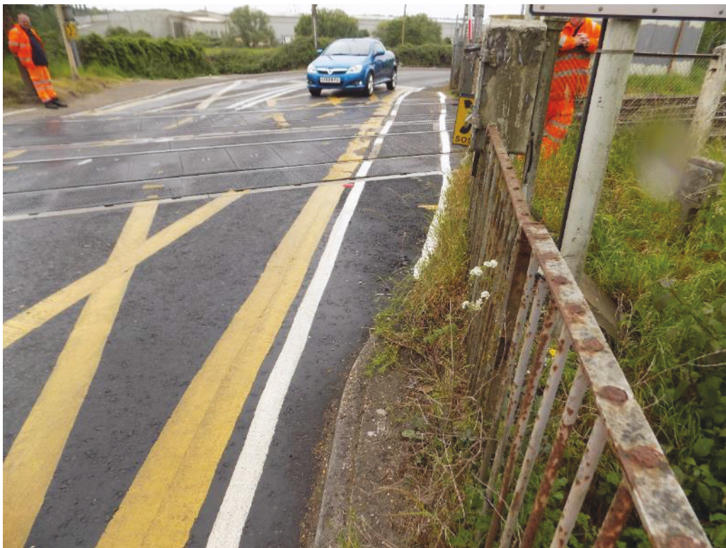
Figure 2-7 - Footway over Crossing (West Side) - Note No Adjoining Footpath at ZO Corner
