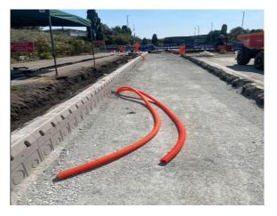
Carriageway backfilled to Type 1 level.
