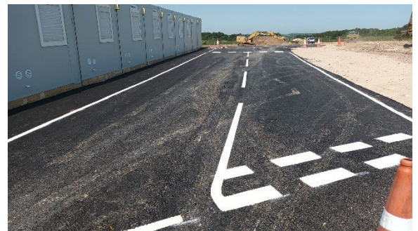
Image: New Temporary Compound in Section 2B
