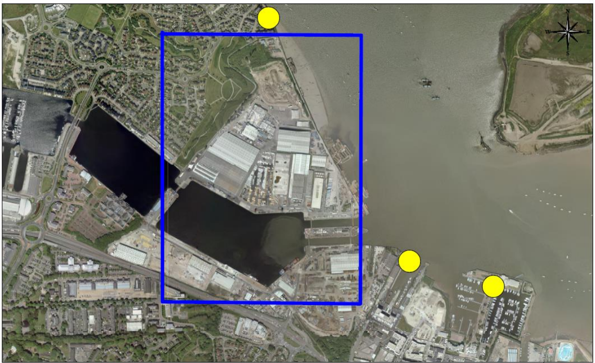
Zone 3 including access points - Aerial view
